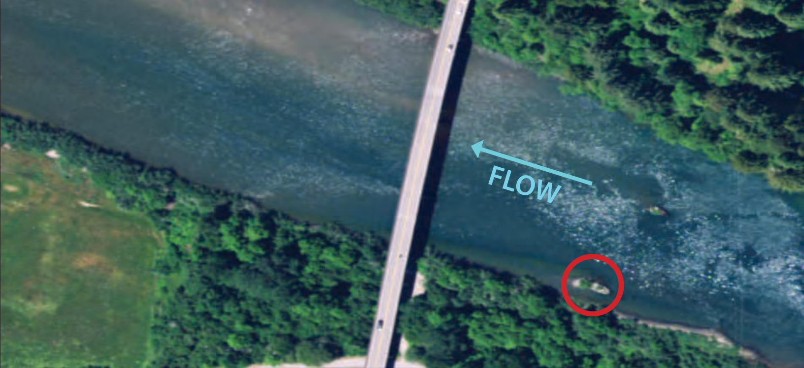
Figure 21. A bridge once crossed this river to the right of the existing bridge. The old concrete piling circled in red was left in place and created a sheltered area along the bank (note the relative smoothness of the river downstream of the piling) where thousands of western pearlshell are now found. This feature mimics other hydraulic controls upriver, like bedrock outcrops, where the species is also found.
