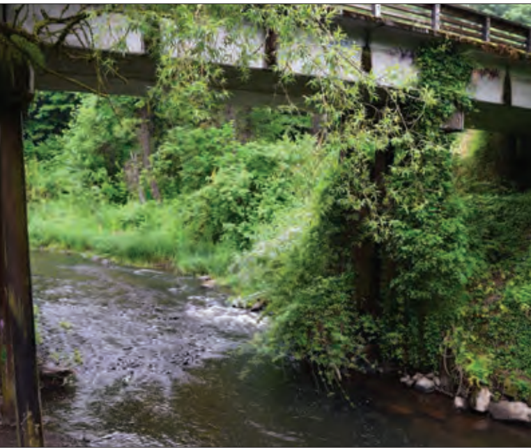
Figure 19. Bridge footings that span streams reduce the need for riprap, as seen along the right bank, that makes for poor mussel habitat unless sediment readily accumulates.
