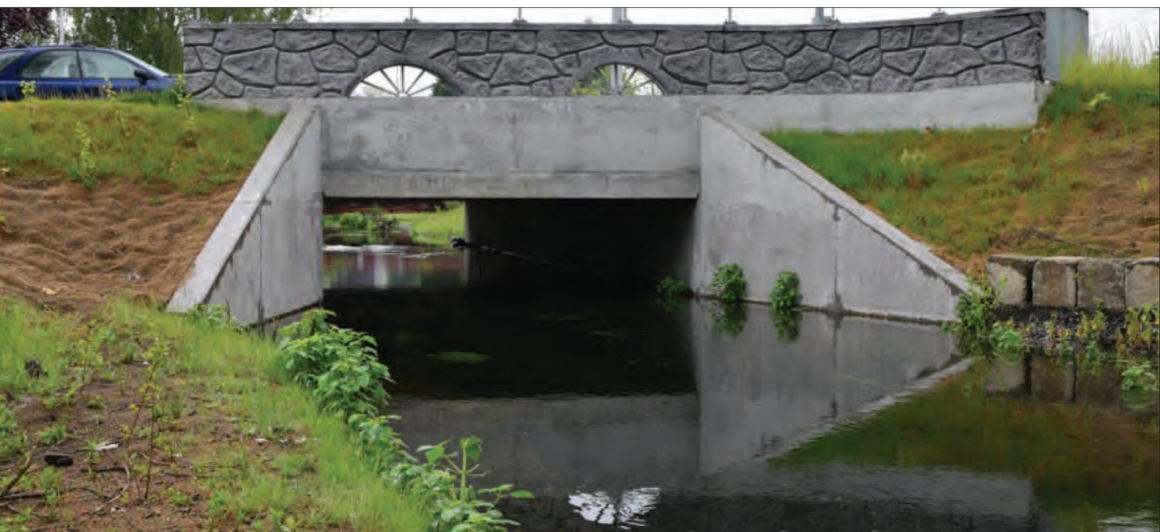
Figure 18. This broad culvert replaced an older, narrower culvert, and was one of several similar projects intended to improve fish passage in a single creek. Floater mussels were found upstream of the old culvert, and a salvage and relocation effort was conducted by Xerces Society and agency staff, as well as volunteers, before construction began. Mussels were also salvaged during the fish salvage and dewatering phases. The group effort ensured that more than 3,000 mussels were saved.
