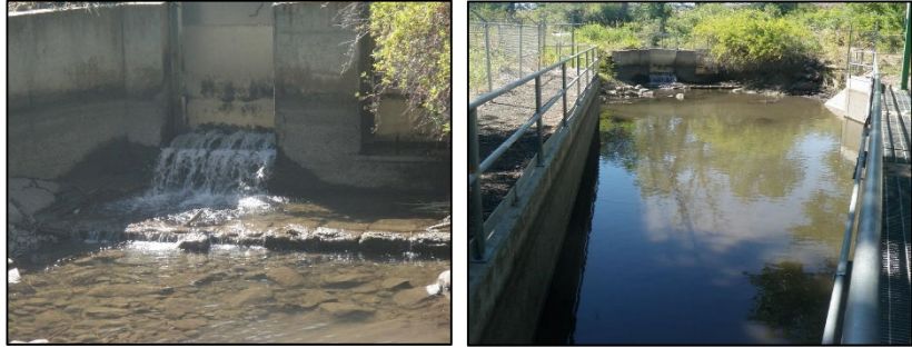
Figure 2. The post irrigation water (~150 gallons min -1 ) entering the area upstream of the headgate (left photo) and the overall wetted area upstream of the fish screens receiving this water (right photo).
