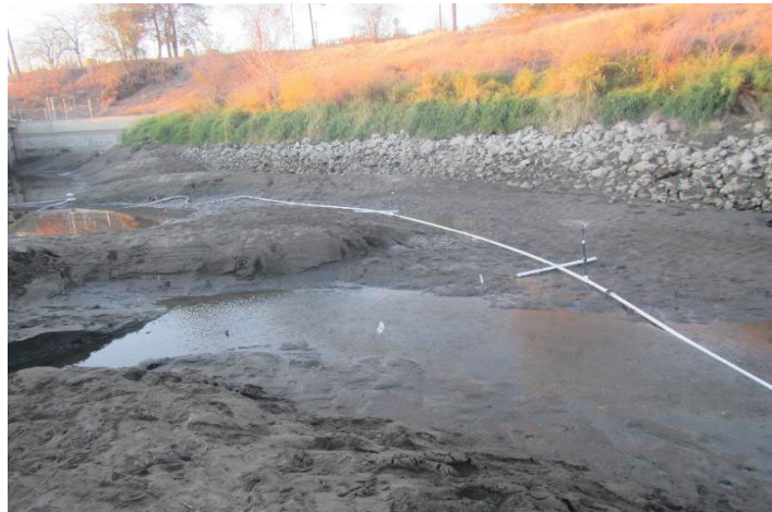
Figure 3. Overview of the sprinkler system operation downstream of the fish screens at Sunnyside Diversion immediately after dewatering of the key larval lamprey habitat occurred. Part of the sprinkler system was able to cover the high density isolated pools.
