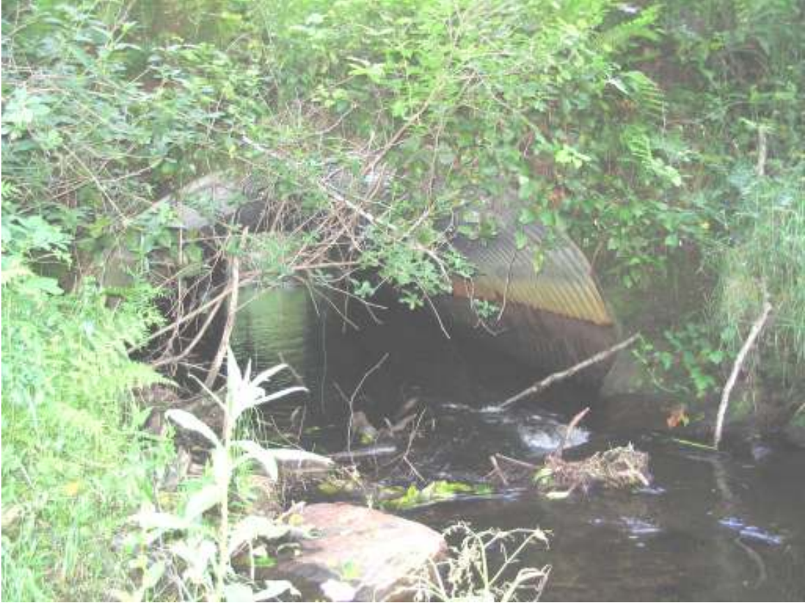
Photo 20. SF Big Cr: Culvert at Blodget Rd crossing.
