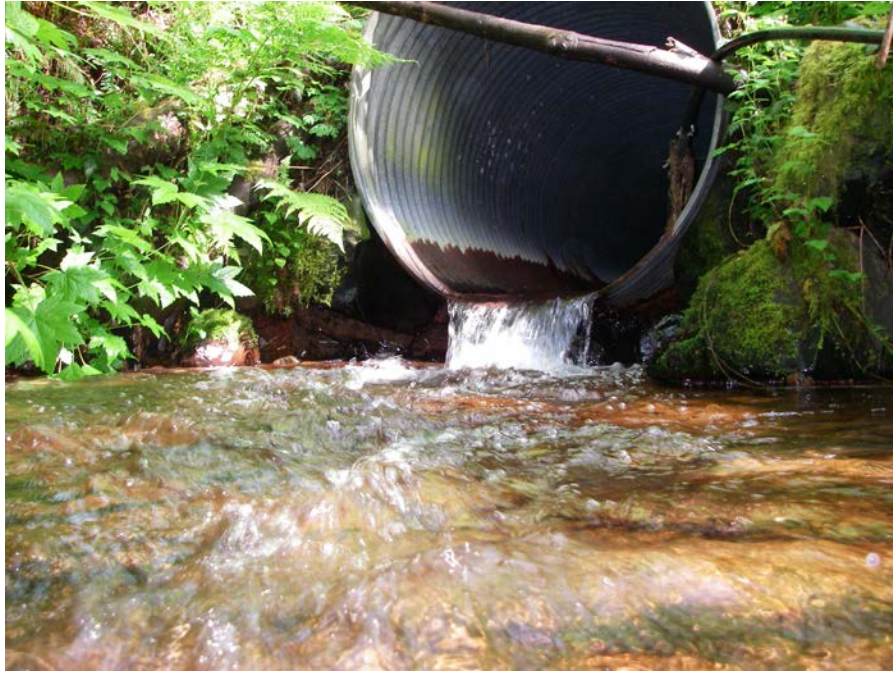
Photo 4. Second Bryant Creek culvert juvenile barrier
