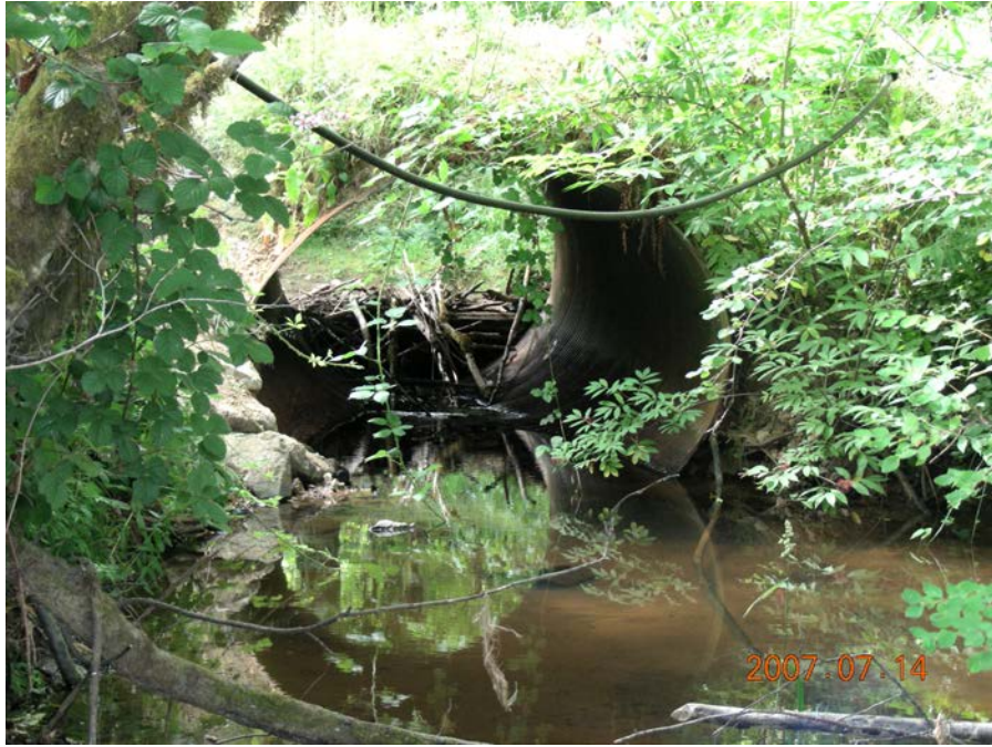
Photo 13. First pipe on Spilde Creek
