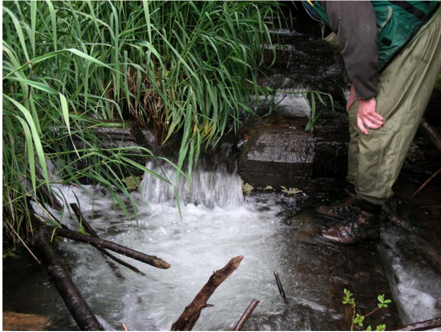
Photo 5. Stony Creek juvenile barrier at county road culvert
