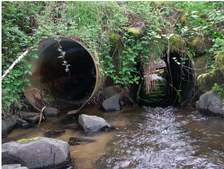
Photo 1. Double culvert on Buttermilk Creek
