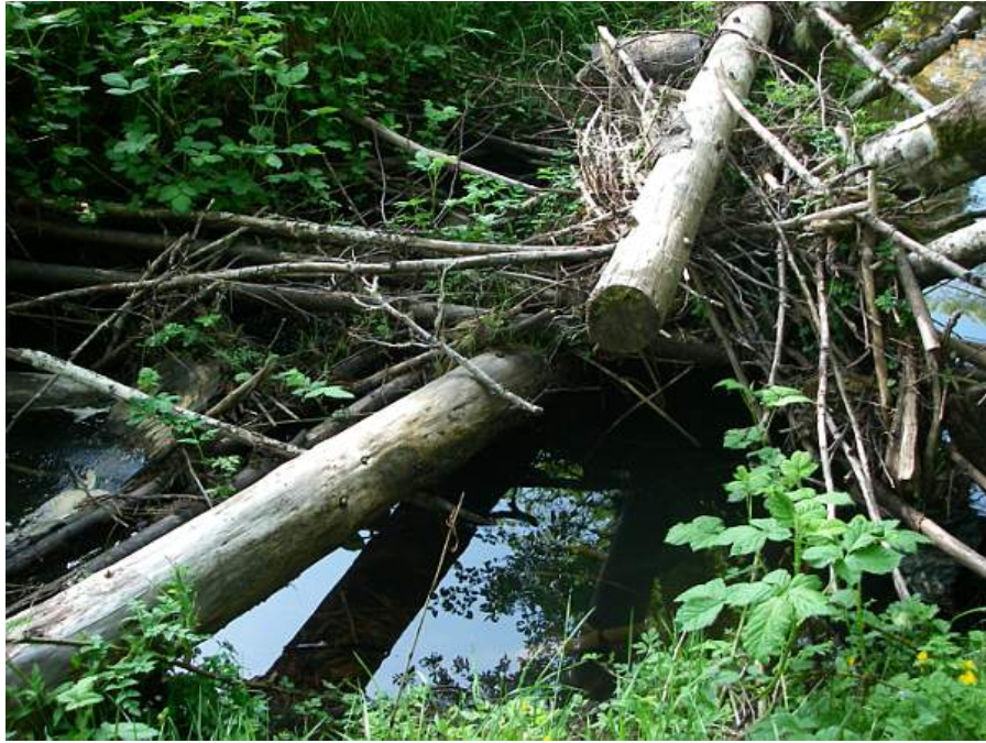
Photo 11. Highly functional Structure on Humphrey Creek illustrates value of small wood in structure design
