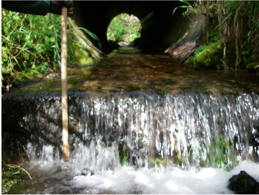
Photo 3. Juvenile Barrier at county road culvert Bryant Creek
