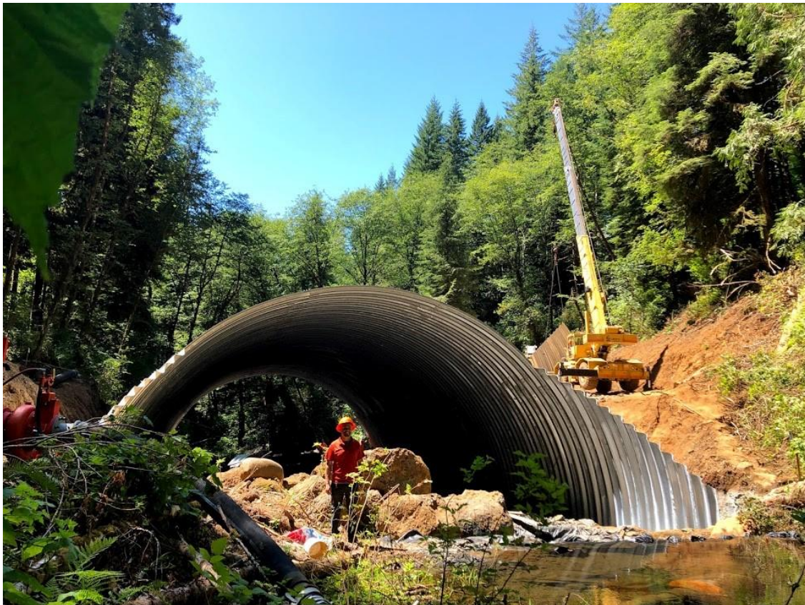
Forest Supervisor Robert Sanchez provides scale for the huge new culvert.
