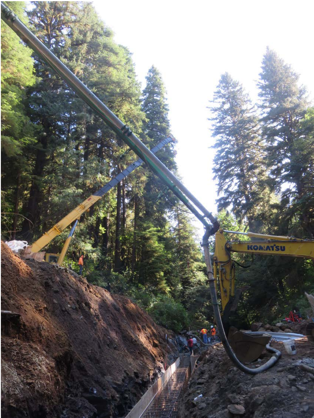
Pump truck set up to deliver concrete to the footing.
