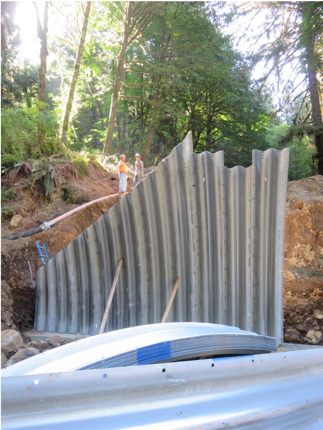
First panels of new culvert installed, it is gonna be huge!
