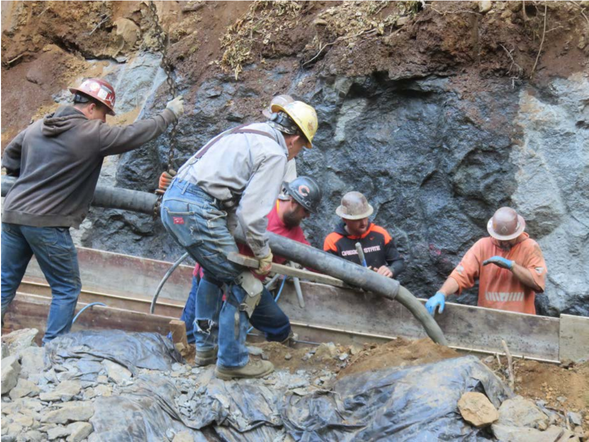
Footing pour #2 (Wednesday, July 24 th ):
